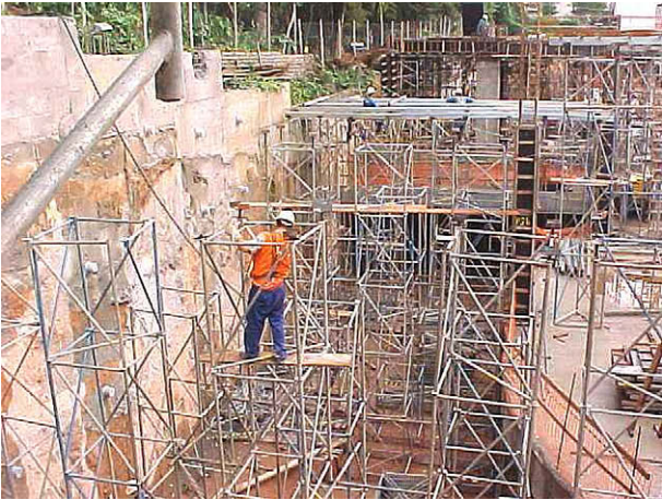
Fig. 3. Activity of mounting and dismantling shoring towers which generated near misses with both positive and negative feedback.
